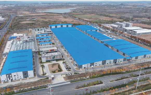
Aeroview of Chuzhou Storage Factory
