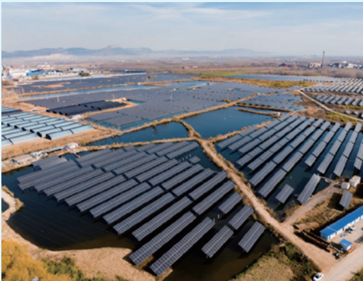
The aquavoltaic solar-storage project in Feicheng city, Shandong province
